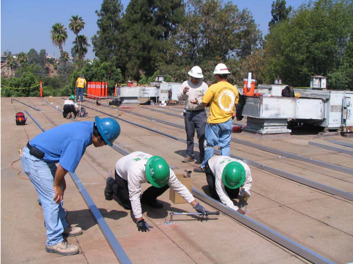
Corpsmembers at Obregon Park
