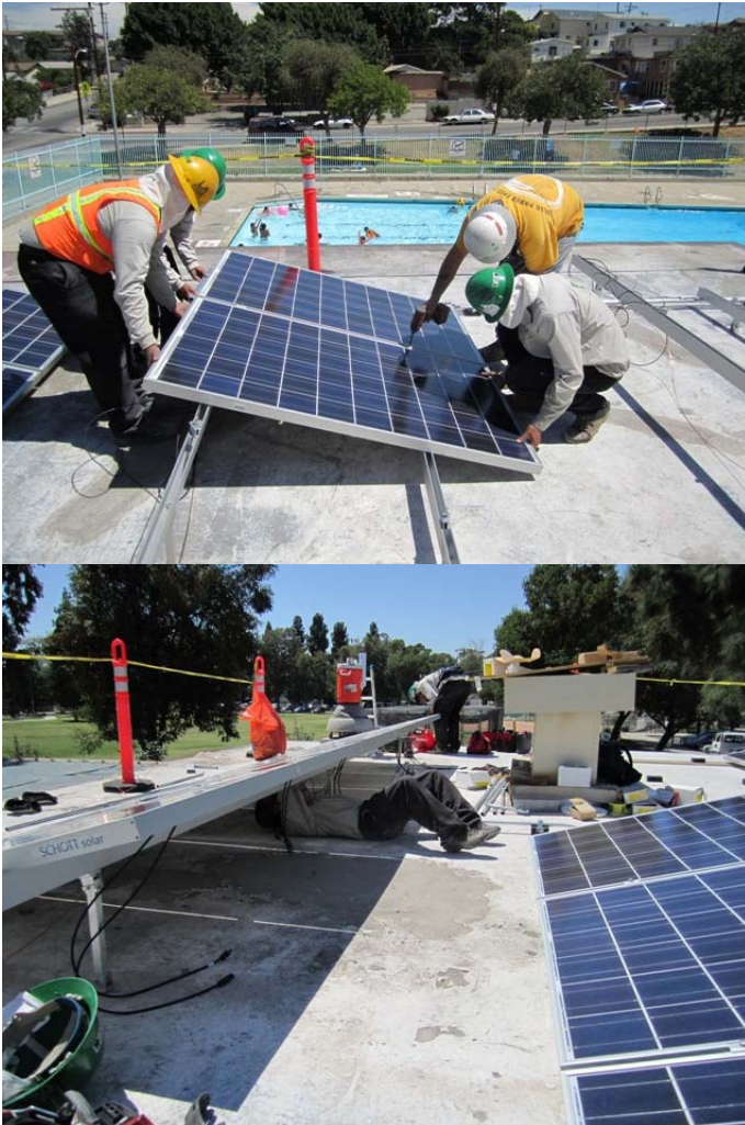
Corpsmembers install photovoltaic panels at Obregon Park
