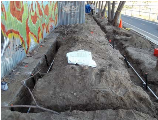
This is the irrigation that the crew has installed
