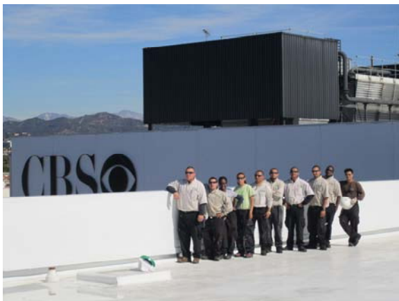
Corpsmembers on the Solar Panel Installation crew at their new job site
