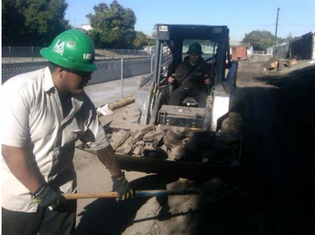
Corpsmembers working on asphalt removal at Compton Creek
