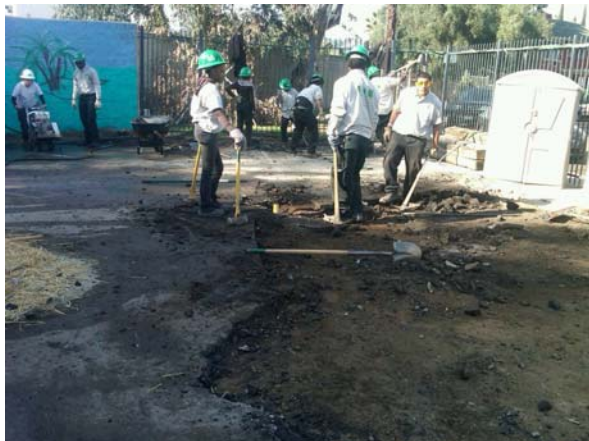
Corpsmembers clearing way for a new garden
