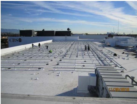
Corpsmembers on the main studio building constructing the racking system.
