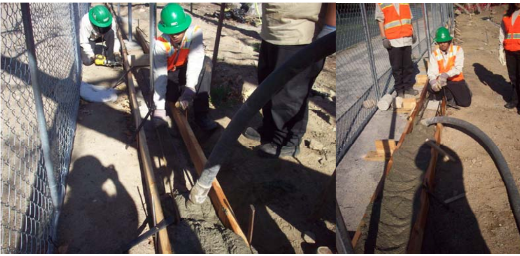
Corpsmembers pouring concrete curbs
