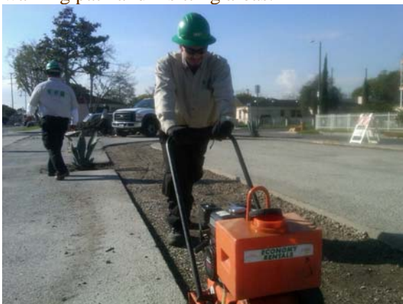
Corpsmembers cleared asphalt to make way for a walking path
