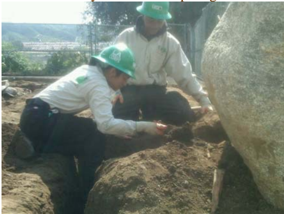
Corpsmembers installing the irrigation system at the El Cariso smart garden
