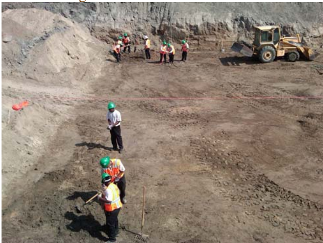
Corpsmembers at Compton Park prepping CMP pipes for installation
