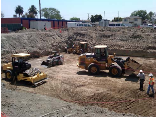
Crews preparing for the sub-grade inspection
