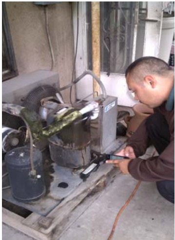
Corpsmember Moises Robledo entering the horsepower of the compressor into the iPhone energy survey
