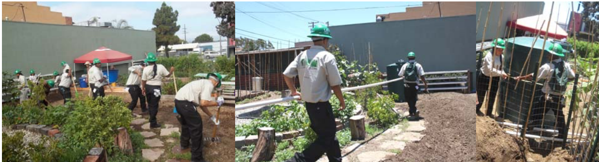
Corpsmembers work on bioswale and installing rain barrel
