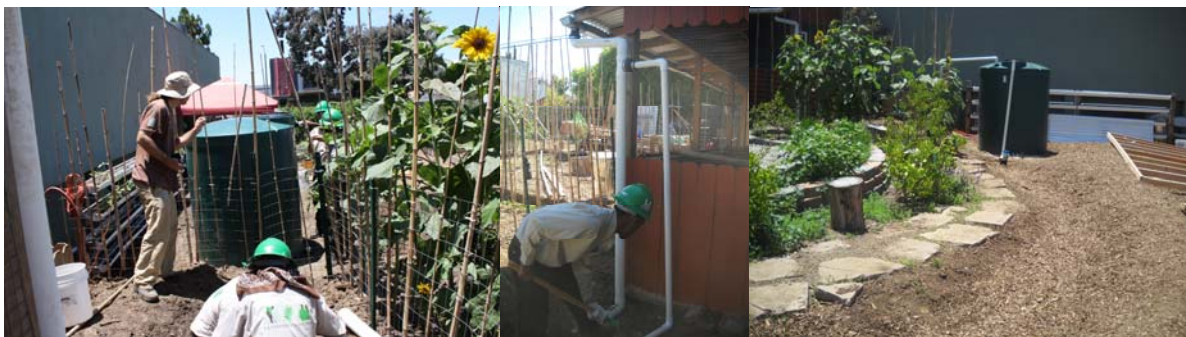
Jeff Adams from ARCSA gives corpsmembers directions on installing the pipes
